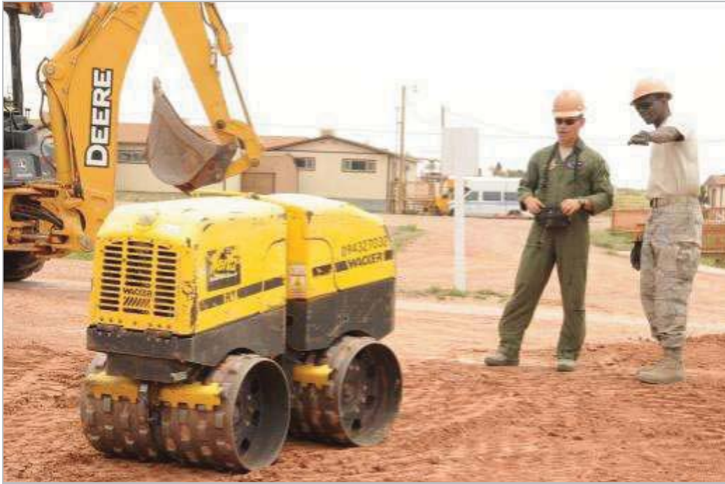
Staff Sgt. Mustafaa White, equipment operator, 113th Civil Engineer Squadron, District of Columbia Air National Guard, shows Brig. Gen. Jefferey Johnson, 113th Wing Commander, how to use a 'sheeps foot roller' to compact dirt during a humanitarian project in Window Rock, Ariz., June 2, 2011. Members of the 113th CES are in Window Rock, Az., as part of the Innovative Readiness Training, a civil-military affairs program linking military units with civilian communities for humanitarian projects. (U.S. Air Force Photo by Tech Sgt. Craig Clapper)
